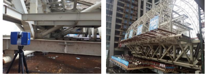
Figure 4. Scan the ground lifting section and its ends
